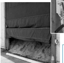
tracks. They used materials from the shop: truck tarps, fence top rail, cable, hardware, and a winch. The second door cost about a quarter what the commercial one for the dome had cost.
