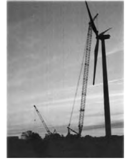
Wind farm tower construction.
