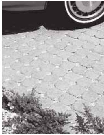
Pervious concrete pavers
