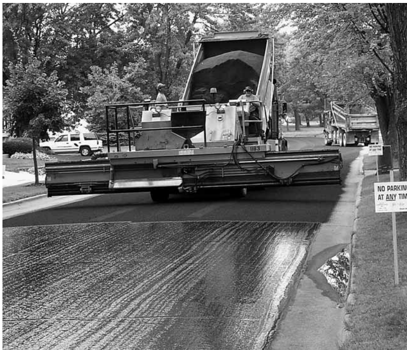
Regular chip seal treatments can almost double the life of a residential street. Good information and some extra sweeping can secure acceptance.
