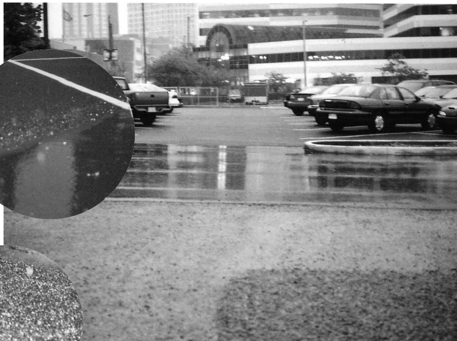
Rain water drains through porous asphalt top and bottom, but remains on standard asphalt (center).
