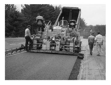
Adding polymers raises the cost of the binder. Although it varies depending on the selected range, WisDOT has been paying \$30-\$70 more per ton of liquid asphalt for polymers on top of about \$160 per ton for unmodified (or natural) binder. To save money, Brokaw recommends using an unmodified binder on the lower layer because the maximum temperatures stay cooler and minimums don't get as cold in that layer.
