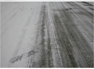
Photos taken during an anti-icing pilot De Pere conducted two years ago show the contrast between the brine-treated half of a city street on the right and the untreated side. Application at the onset of a storm helped break the bond of snow and ice to pavement, making clean removal easier.
