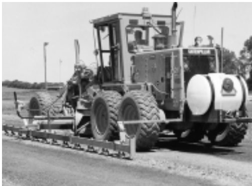
Injecting foamed asphalt during pulverizing shows promise (far left).
