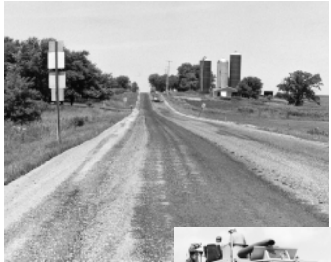
Reclaiming uses old asphalt pavement to strengthen the road.
