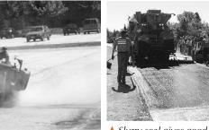
▲ Slurry seal gives good surface protection and appearance of new road surface.
