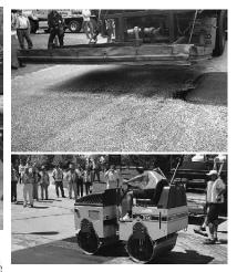
Infrared patching and rolling provide excellent appearance, a smooth ride, and long lasting patches.
