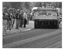
▲ Chip seals provide cost effective preservative treatment. Calibrated equipment and trained crews are required. Pre-coated chips limit dust and give a new asphalt surface appearance.
