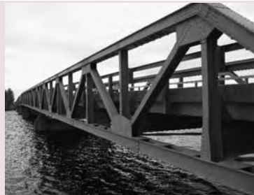
The six-span steel truss CTH M Bridge over the Chippewa River has a new load rating and posting BELOW after a review in 2007.
