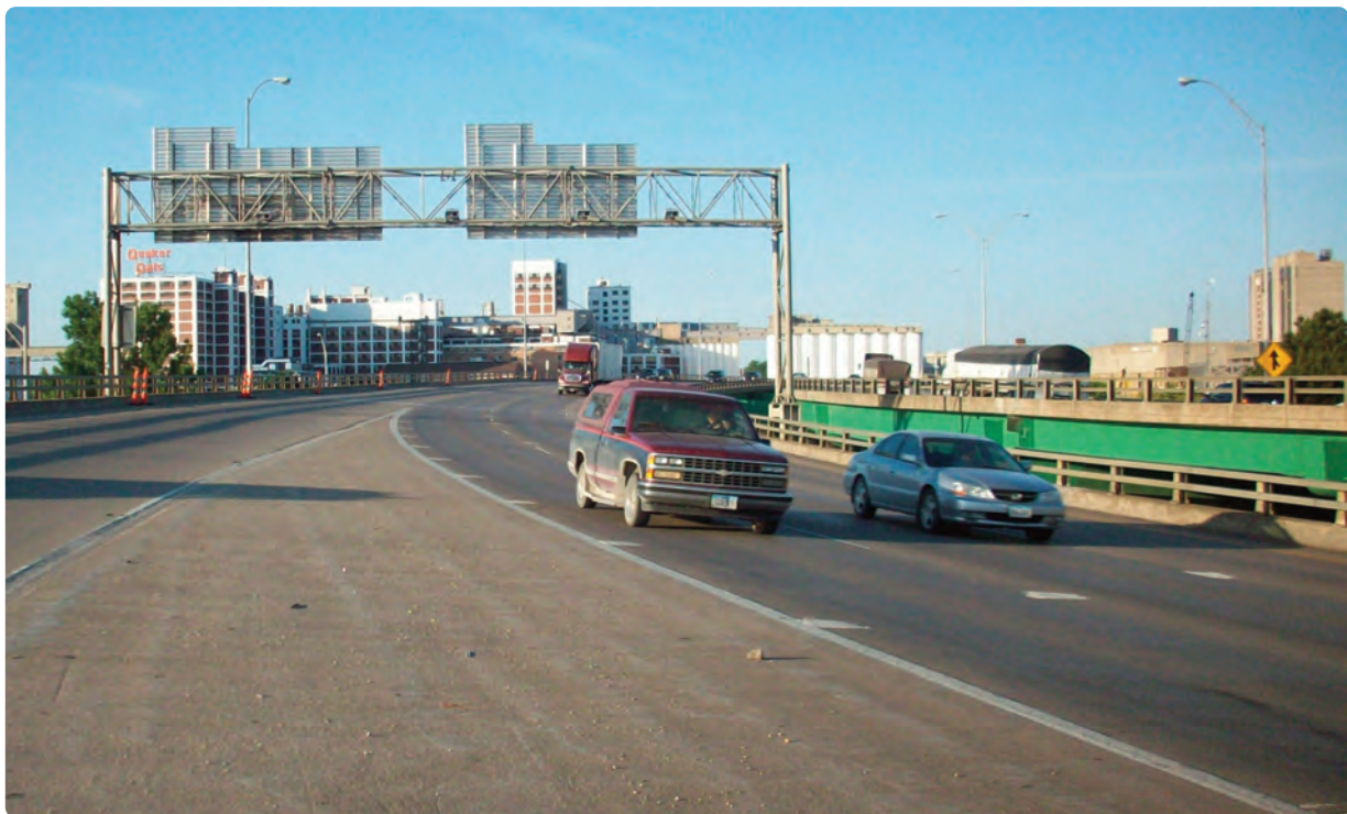
The curve of the road, traffic volumes and its crash history made the Cedar Rapids highway bridge a good candidate for the high friction surface treatment the Iowa DOT installed in 2012.
