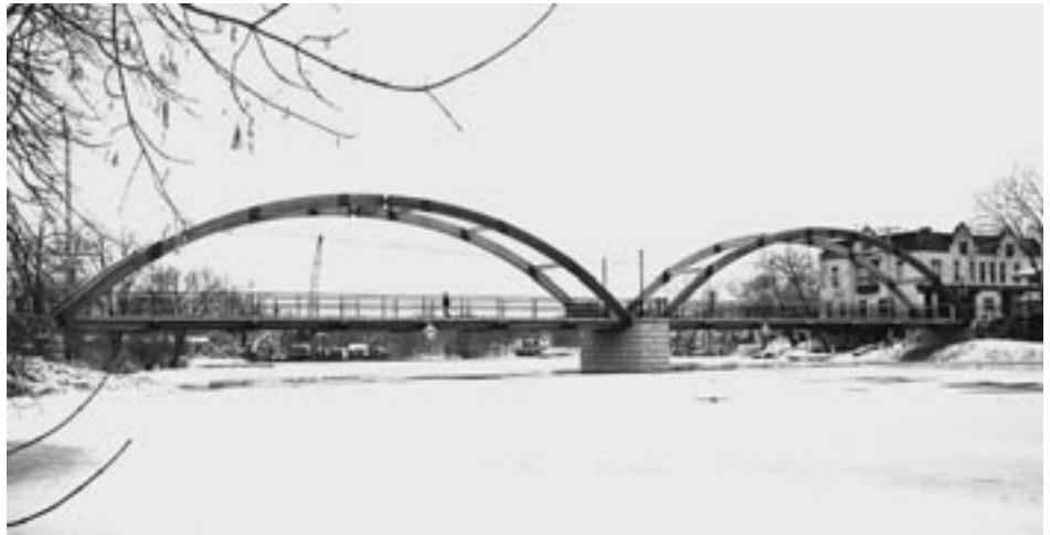
This new bicycle/pedestrian bridge crosses the Rock River in Jefferson.
