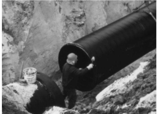
Lighter weight and lower cost make plastic pipe attractive for storm drains and culverts.
