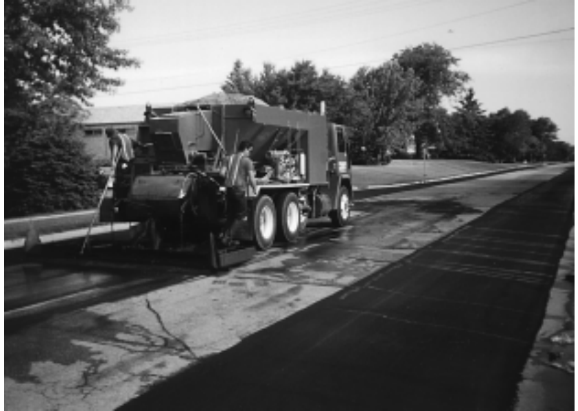
Sealcoats are keeping some Sun Prairie streets from getting worse. Roadware helps select the streets and shows the payoffs.
