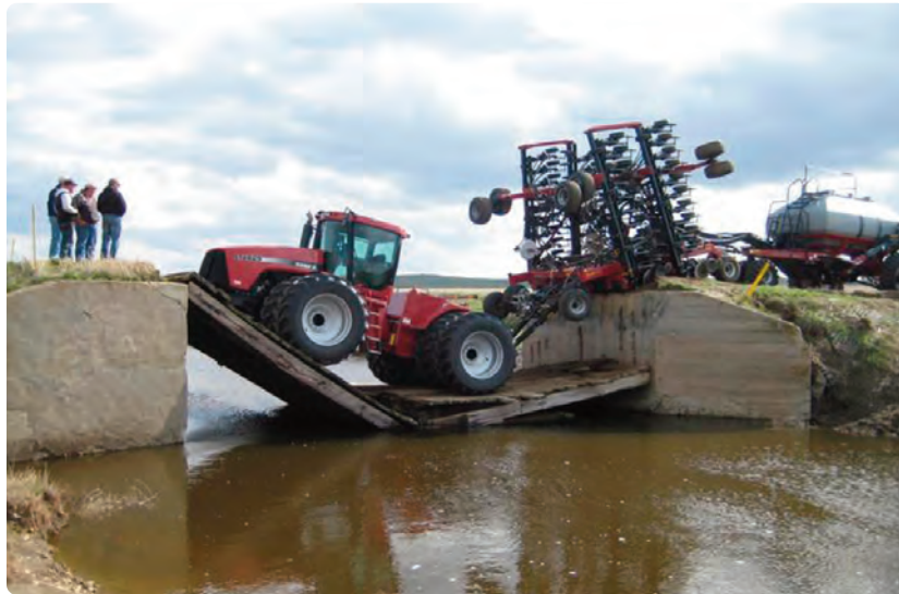
Consequences of bigger, heavier, wider ag equipment traveling on local roads include tangling with utility poles and wires, damage to pavements and causing a bridge collapse. Local governments try to intercept potential problems through a range of best practices that serve the public and meet the needs of commerce.
