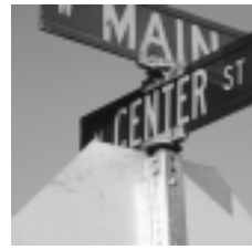
Mounting unrelated street signs with stop signs is against MUTCD guidelines. This is now being reconsidered.
