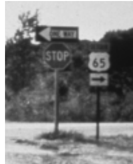
Unrelated arrow sign is incorrectly mounted with stop sign (left). Good sign installation with route marker separate from stop sign and supplemental sign mounted below it (right).
