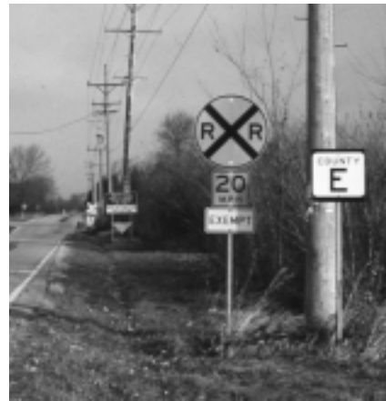
Railroad exempt signs, authorized only by WisDOT, inform school bus drivers and others that they are only required to stop if a train is approaching.
