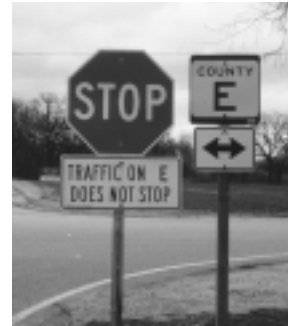
Unrelated arrow sign is incorrectly mounted with stop sign (left). Good sign installation with route marker separate from stop sign and supplemental sign mounted below it (right).
