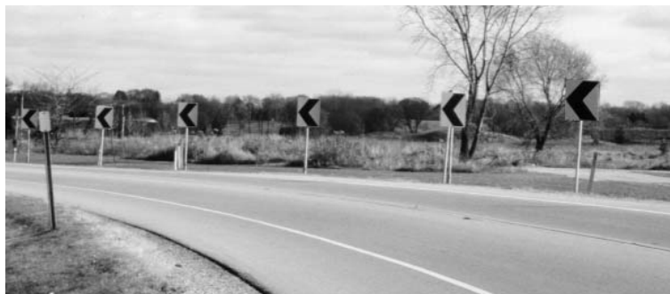
Improved signing on curves and turns cut crashes 34% in Mendicino County.
