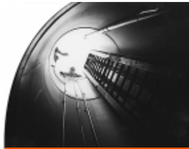
Confined spaces, like this underground tank, are one of 11 topics offered at safety seminars this fall.
