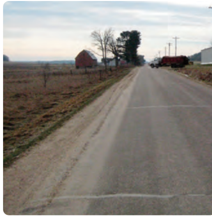
Lincoln Road in Jackson County shows serious deterioration along its entire 3.4 miles, a major reason the Town of Curran applied for TRID funds to upgrade it. Curran shares costs with the Town of Springfield of rehabilitating the pavement, adding a gravel shoulder and widening driveways where heavy farm equipment travels and turns.
