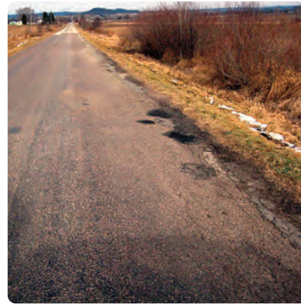
Lincoln Road in Jackson County shows serious deterioration along its entire 3.4 miles, a major reason the Town of Curran applied for TRID funds to upgrade it. Curran shares costs with the Town of Springfield of rehabilitating the pavement, adding a gravel shoulder and widening driveways where heavy farm equipment travels and turns.
