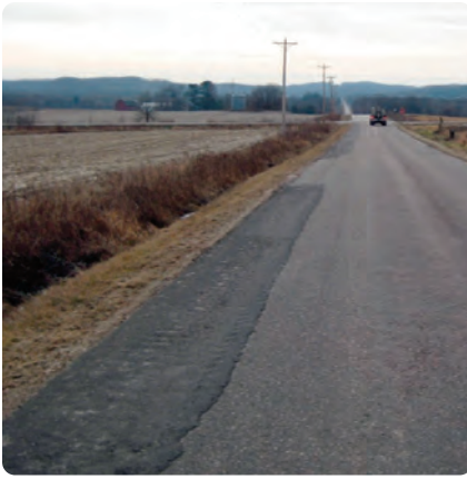
Lincoln Road in Jackson County shows serious deterioration along its entire 3.4 miles, a major reason the Town of Curran applied for TRID funds to upgrade it. Curran shares costs with the Town of Springfield of rehabilitating the pavement, adding a gravel shoulder and widening driveways where heavy farm equipment travels and turns.
