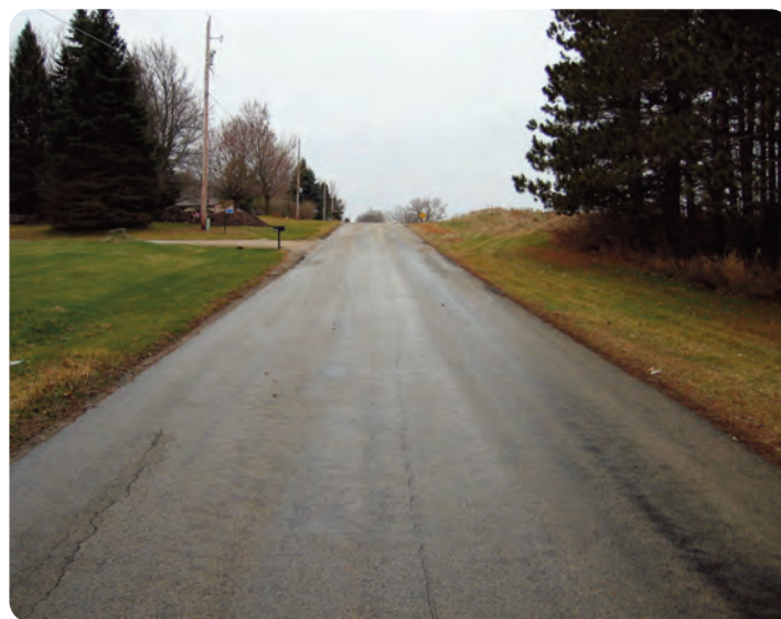
Main Road in the Town of Ellington carries up to 2,100 vehicles a day on narrow pavements with no shoulders and vertical curves that affect sight distances. It is getting a much-needed upgrade this year thanks to TRID funding.
