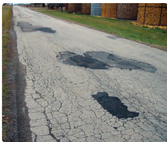
The Town of Ellington project reconditions a substandard road with cracks, potholes and patched areas that make it a rough road to travel. Now as narrow as 16 feet in some places, TRID-funded changes will widen it to 22 feet and add a four-foot, partially paved shoulder.
