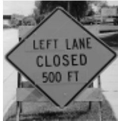
The A-frame barricade and rigid sign do not meet the new crashworthy requirements.
