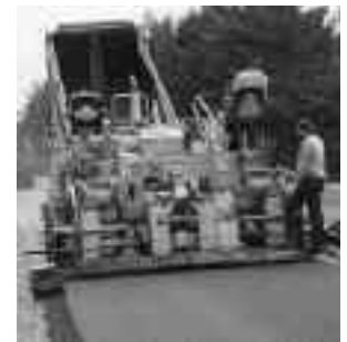
Upgrading decisions usually involve safety, quality of life and other factors.
