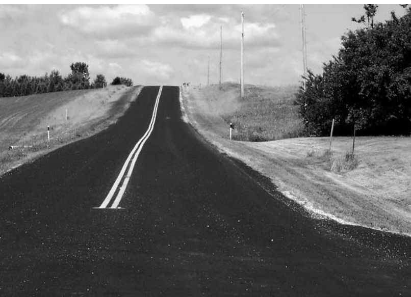
After betterment. Shoulders wide and flat. Utility poles moved back.
