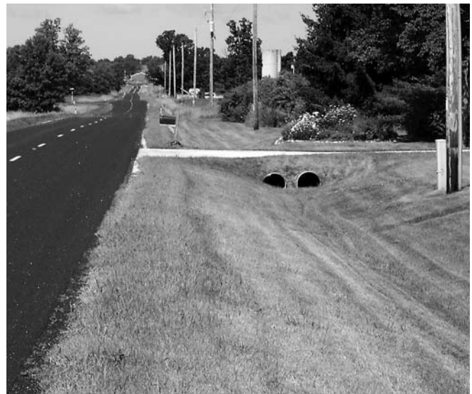
New driveway culverts benefit landowners as well as town road.
