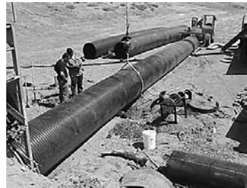
Traffic, utilities, and pavement are undisturbed with sliplining
