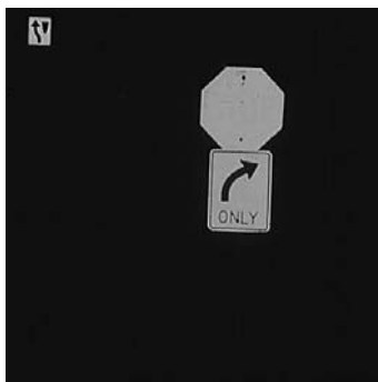
Use regular nighttime inspection to find failing signs like this.
