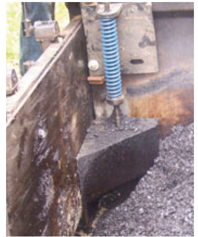
Trans Tech shoe attached to paving screed creates the Safety Edge.
