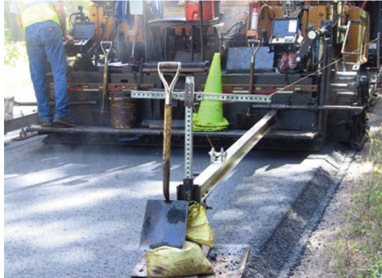
Paver advances on the STH 55 project, producing the Safety Edge as it goes.
