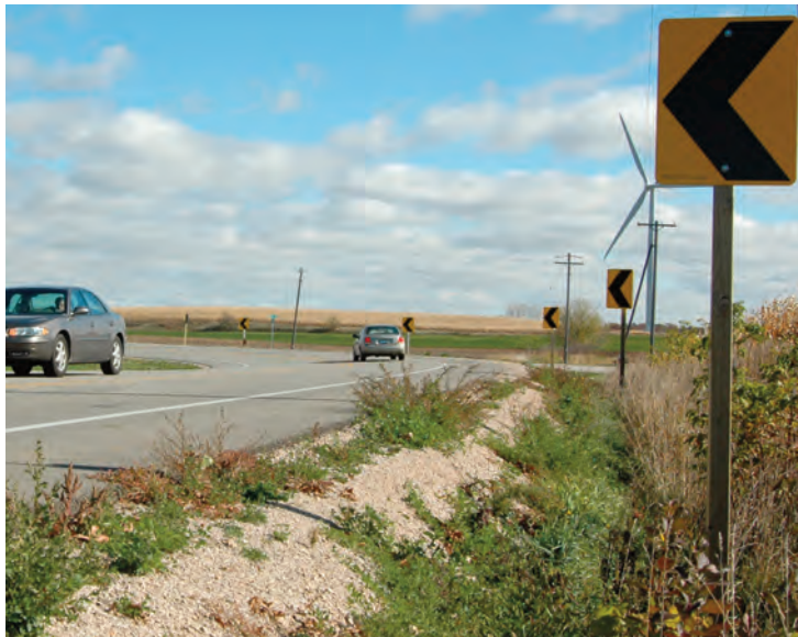
Close up of a Fond du Lac County spot map (top) shows the location of single-vehicle crashes along a tight curve. The visual data helped the county prioritize cost-effective safety measures as part of a resurfacing project that included paving shoulders around the curve and installing chevrons, as seen in the photo above.
