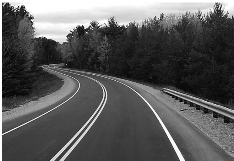
Wilshire Drive in the Town of Hull, improved in 2007, is a listed road under the new ordinance where a weight limit of 15,000 lbs per axle applies.
