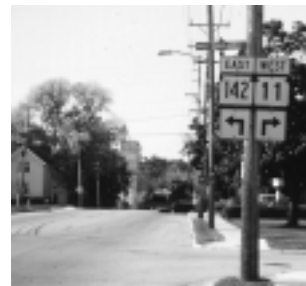
Mounting signs on utility poles requires the owner's permission.
