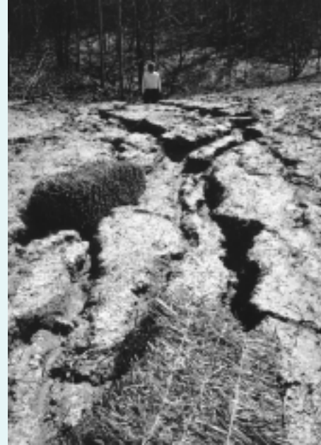
Too little, too late. Plan ahead for erosion control. Have all materials on site before you make the first soil cut. FDM Chapter 10 can tell you how (see Resources pg. 6)
