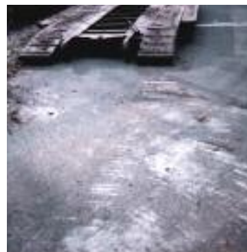
Before and after photos of a town road show the damage done by a contractor unloading heavy equipment. Following permit requirements, the company reimbursed Hull for the cost of repairs.
