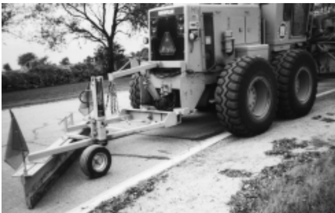
Trailing a second blade eases shoulder repairs
