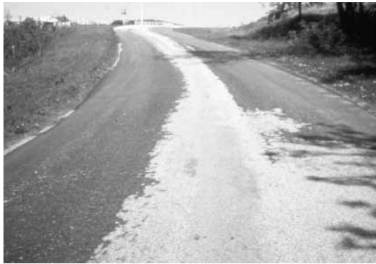
Roads like this rate 5 on PASER's 10-point scale: good structure but needing sealcoat or overlay.
