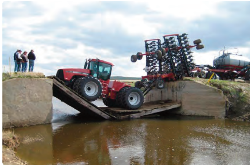
Consequences of bigger, heavier, wider ag equipment traveling on local roads include tangling with utility poles and wires, damage to pavements and causing a bridge collapse. Local governments try to intercept potential problems through a range of best practices that serve the public and meet the needs of commerce.
