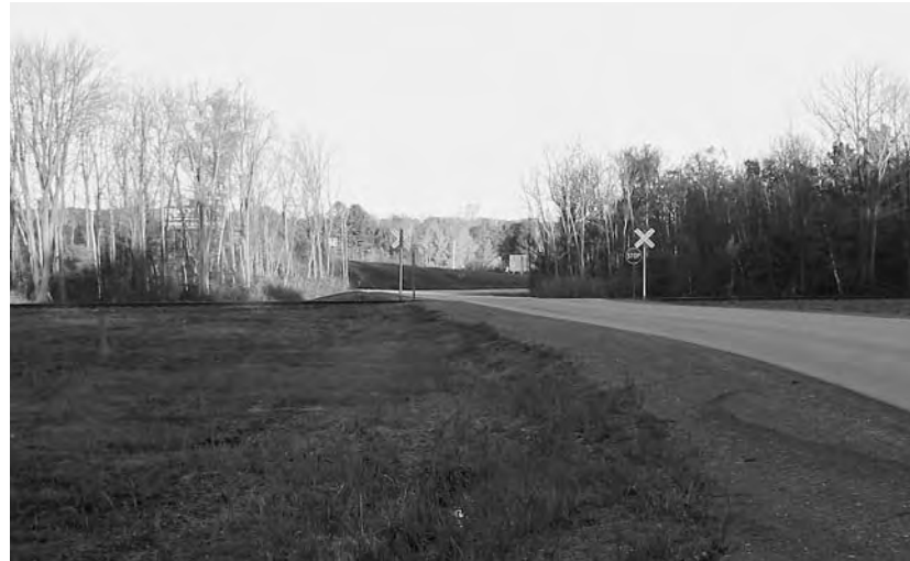
A vision corner at ground level. Clear cutting ensures adequate time for traffic to stop safely.
