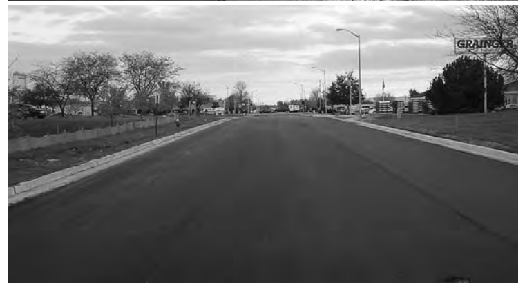
Before ABOVE and after photos of a section of the Northbranch Industrial Park road the City of Oak Creek rehabilitated in 2007 using pulverization. The project also added curb and gutter elements.
