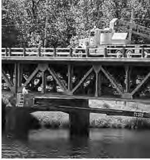
A bridge inspection in progress.
