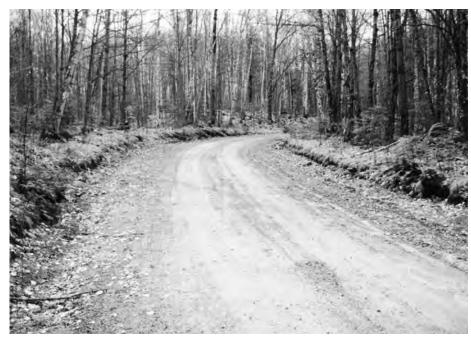
No ditch. Road is actually trenched into roadside forcing water onto surface.
