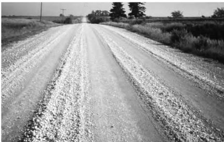
Heavy accumulation of loose gravel requires regrading. Ditch cleaning needed on right side.
