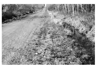
▲ Lack of ditch on right causes ruts. Needs gravel.
