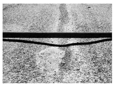
Rut in wheel path needs regrading to eliminate ponding and prevent further road deterioration.
