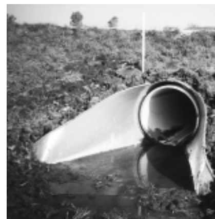
Plastic liners have higher flow rates than corrugated metal. Grout fills the cavity between liner and culvert.
