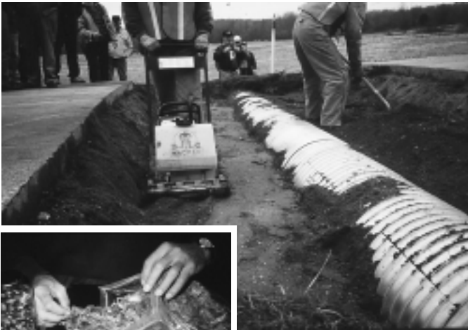
Unwanted glass is easily disposed in culvert fill base course or cold mix asphalt.
