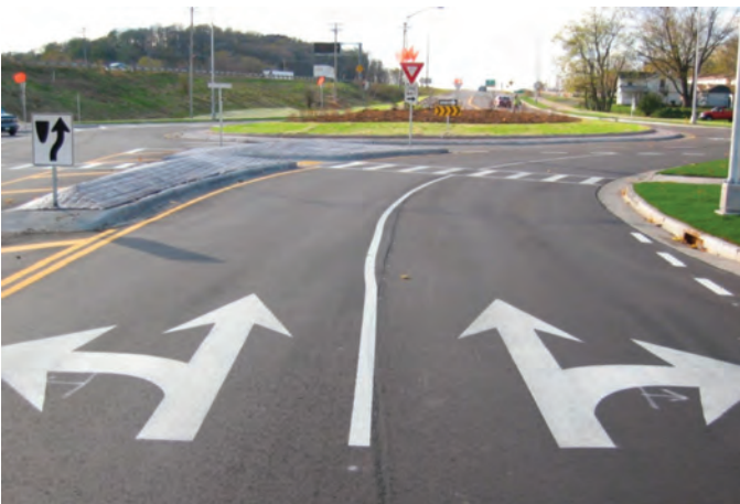
Two examples of entry lanes in a two-lane roundabout. At left, pavement markings guide drivers' lane choice and, at right, a gore area between lanes gives large trucks room to maneuver safely into the circle.
