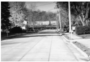
A thin layer of concrete can rehabilitate asphalt pavement. The resulting rigid pavement can be especially useful at intersections with high levels of traffic-related surface damage.
