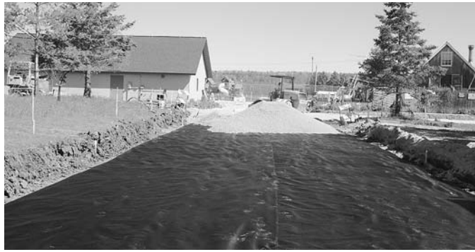
Using geotextile fabric over bad soils, like this clay on Madeleine Island, saves money and makes a better road.
