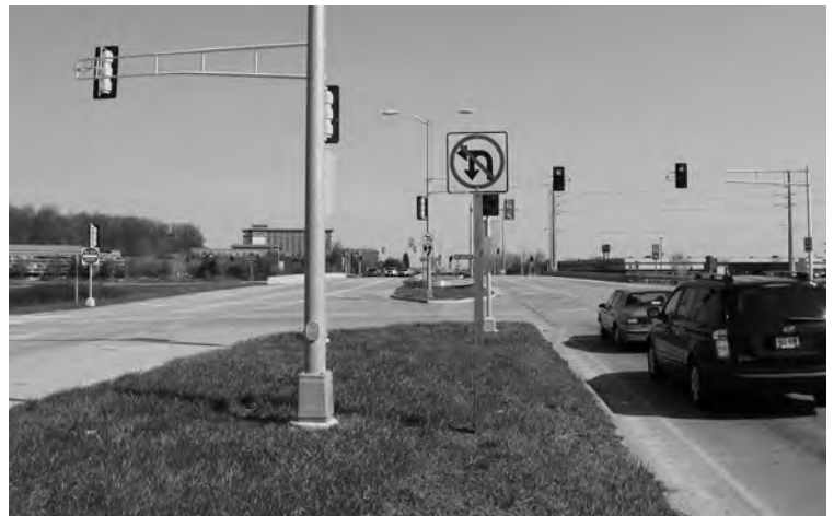
Sign in median prohibits both U-turns and left turns at intersection on a divided highway.
