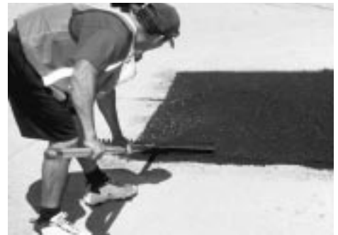
It is important to be clear in bid documents who will do patching and repairs before the sealcoat or overlay is applied.
