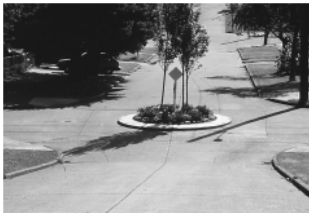
Traffic circles slow traffic, beautify residential streets and allow service vehicles to pass easily.
