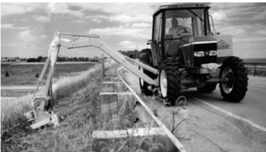
A mower mounted on an arm helps maintain vegetation behind guardrail.
