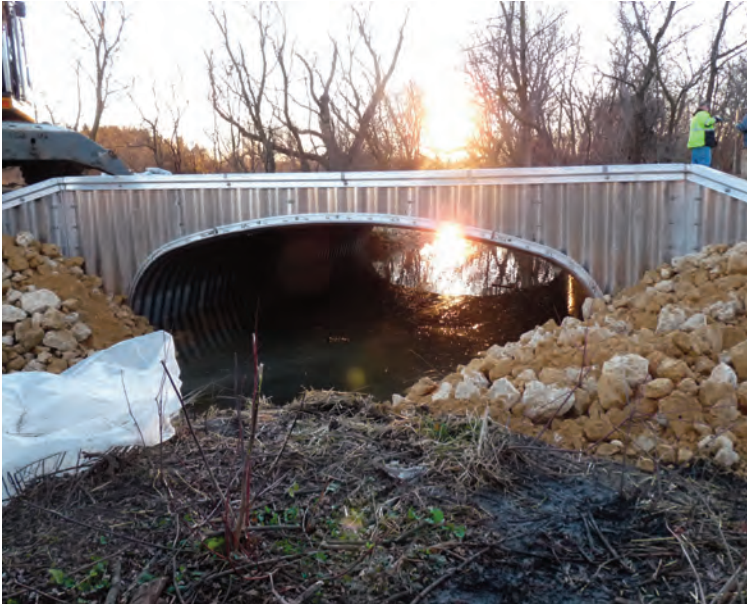
LEFT: The new bridge takes shape on day six with abutments in place and a rebuilt stream bank below. TOP RIGHT: The completed aluminum culvert bridge seen from below with stream flow restored and new guardrail in place. BOTTOM RIGHT: A view from the bridge approach to the new asphalt pavement.
