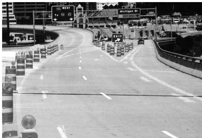
Setting up work zones takes the right equipment, judgement, and inspection.
