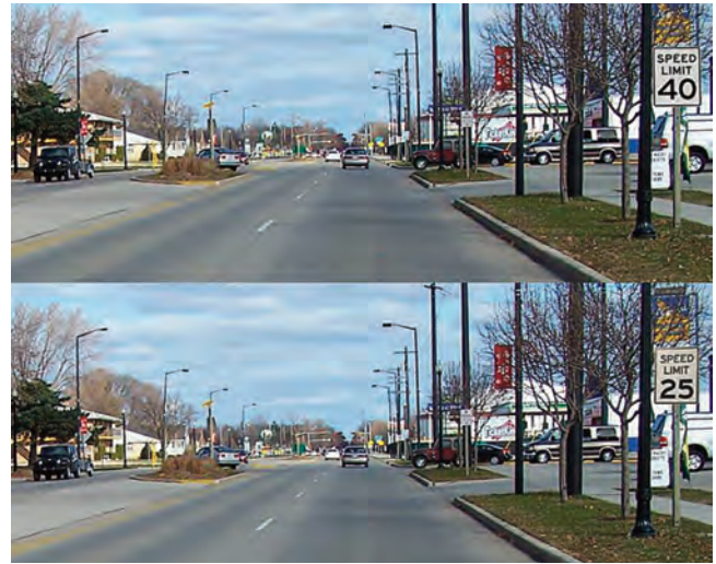
Which speed is the rational speed? Two versions of the same photo illustrate road characteristics, like four travel lanes divided by medians on a mostly commercial roadway, that factor into deciding the answer to that question on this corridor is 40 mph. Taken from a statewide study comparing the safety impacts of rational and irrational speed limits that analyzed the difference between posted speeds and actual speeds on a variety of roads across Wisconsin.
