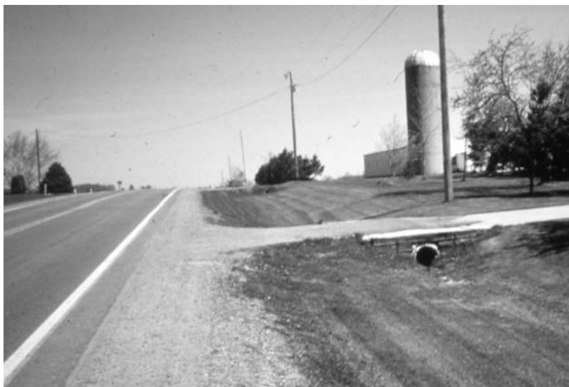
Manage driveway spacing, numbers, locations, and construction with an effective access control ordinance.
