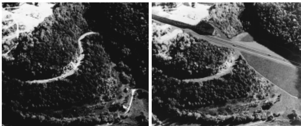
Rebuilding HWY 93 in Trempeleau County was Wisconsin's largest single-season earth moving project ever. The original road is shown on the left; the computer enhanced image of the completed project is on the right.
