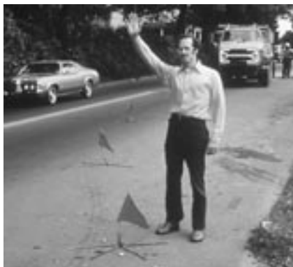
With no safety equipment, flagger is at risk.
