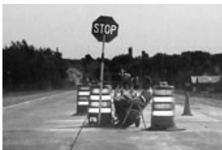
Is this flagger alert to traffic?
