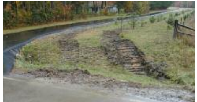
These photos record culvert damage at the entry and exit point after delivery of a heavy load that received a permit to travel on town roads. Such before-and-after evidence helps with enforcement of Hull's weight limit rules.
