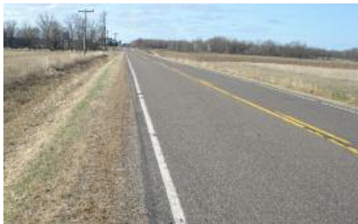
Norby monitored the roads used in the pilot for deposits of salt brine in the spring and found no residue on the pavements test treated during the winter.
