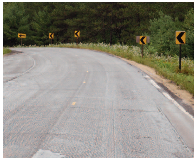
A better position for the large arrow sign at left is in the line of sight for an approaching driver, or about where a chevron is missing in this photo. Another solution on curves like this is to install a series of chevron signs only. Use the MUTCD as a guide for placing road signs correctly.
