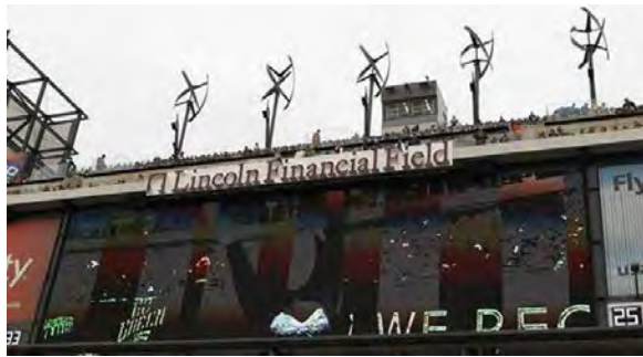
FIGURE 2: VERTICAL AXIS TURBINES LOCATED ON PHILADELPHIA STADIUM (BONDSTK, 2013).
