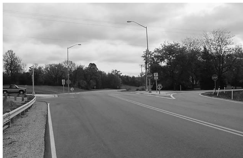
Completed County road (CHIP) project at CTH F and CTH W Intersection in Kenosha County.
